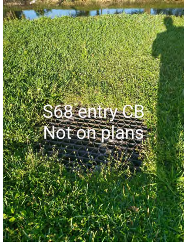
4/5/2022 (S72 Structure, not S68)
