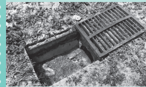
(Top) A stormwater inlet pipe located in a grassed swale is hidden from view due to overgrown vegetation, dirt and leaves. (Center) Proper maintenance should include periodic inspections and removal of excess material and sediment that might block water flow. (Bottom) A clear opening ensures that excess stormwater will properly flow through the drainage system as designed.
