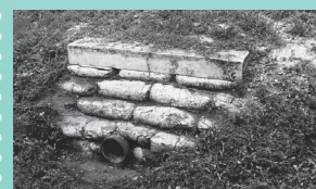
(Top) A stormwater inlet pipe located in a grassed swale is hidden from view due to overgrown vegetation, dirt and leaves. (Center) Proper maintenance should include periodic inspections and removal of excess material and sediment that might block water flow. (Bottom) A clear opening ensures that excess stormwater will properly flow through the drainage system as designed.
